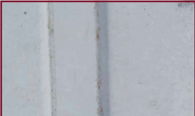
Panel bend corrosion after 21 years
