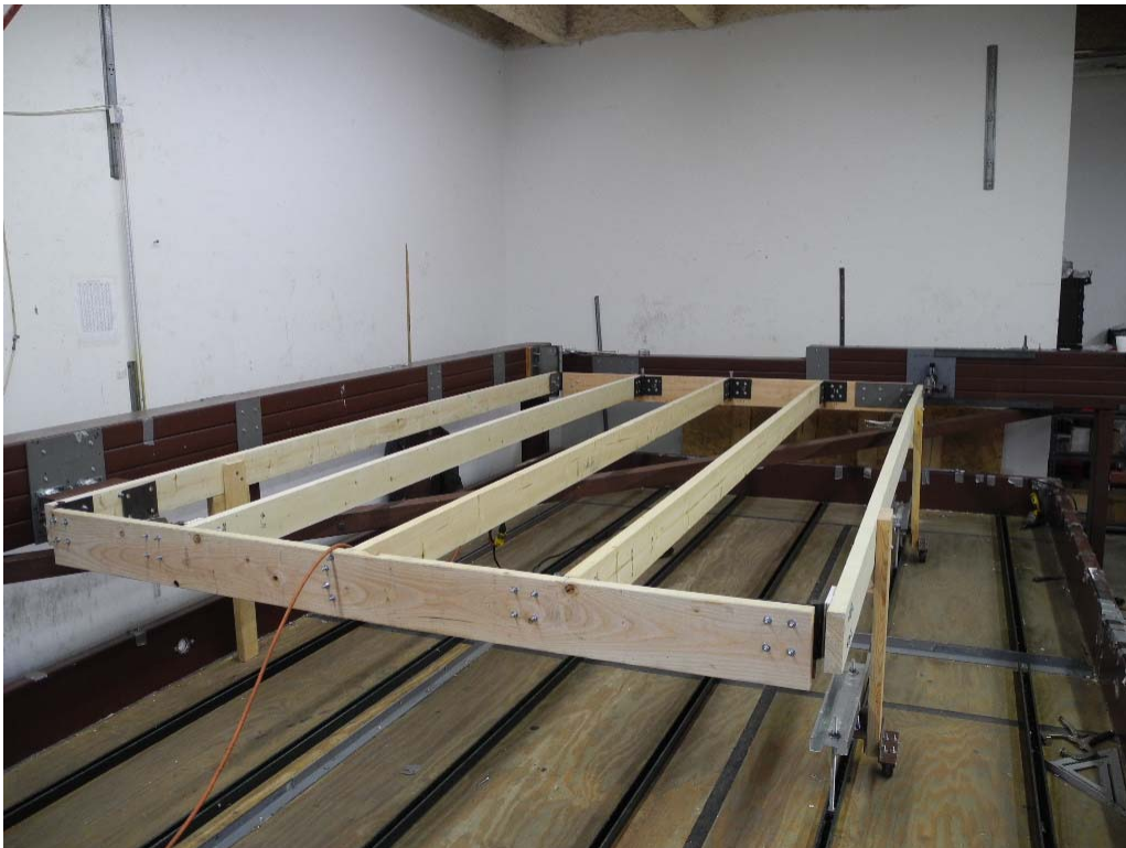
PHOTO 2 View of the wood support layout for panel span of 2' 0". (DSCN0009)
