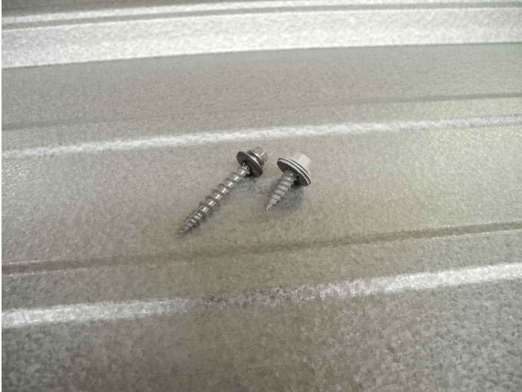
PHOTO 1 View of the structural and sidelap fasteners. (DSCN0005)
